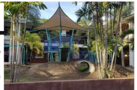
ESTUDIO DAMGO 6 is a grade school playground project constructed in 2017 at Taclobo, Dumaguete City, specifically within the grounds of Foundation Preparatory Academy (FPA). It is near the elementary classrooms, principal's office, and dining area, and is close to university facilities such as a carpentry workshop and a bamboo treatment facility.
