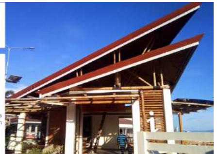
The Tourist Information and Assistance Center is a sustainable project of the Philippine Ports Authority, built in partnership with Foundation University through the Estudio Damgo Team IV. The 72 sq.m. structure is located in Brgy. Looc, Port Area, Dumaguete City, a popular tourist hub. Its purpose is to provide information to tourists on vacation spots, local delicacies, and corresponding pasalubong shops and restaurants.
