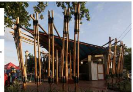
People's Comfort Lounge was a student-led project that aimed to address the lack of public restroom facilities in the south-end of Rizal Boulevard in Dumaguete City, Philippines. The project started with data gathering and design in April 2016 and construction was completed in December 2017 with a budget of Php 1,543,909.75.
